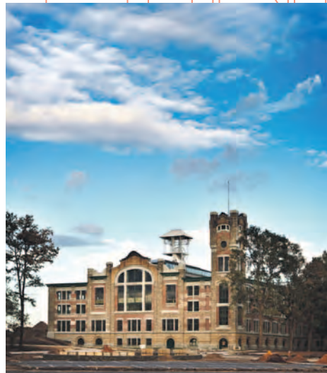
Former coal mine of Waterschei, Genk Photo: Kristof Vrancken
